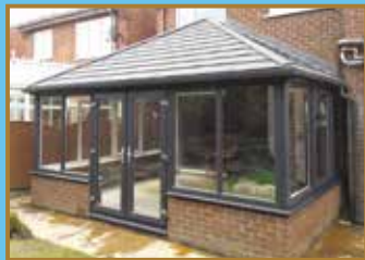
AFTER ROOF INSTALLED
