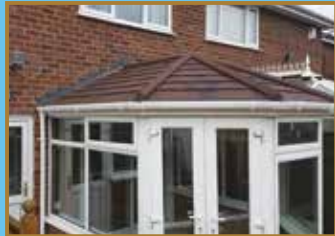
AFTER ROOF INSTALLED
