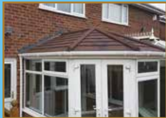
AFTER ROOF INSTALLED
